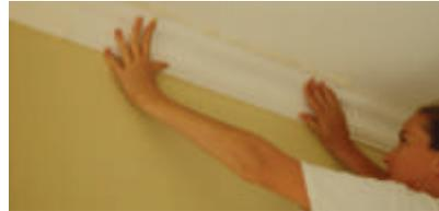
4. Place the cornice on the line and gently press the cornice into place. For joints, apply a small quantity of glue and slide the cornices towards each other to form a closed butt joint.
