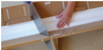
2. Cut (mitre) your cornice to size using a very fine tooth saw.
