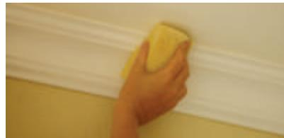
6. With a damp sponge wipe the edges and joints for a perfect smooth finish. Your cornice is now ready to be painted with any water-based paint. No primer is required.
