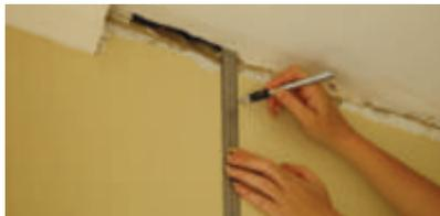
1. Mark the position of the cornice. Draw a line where the cove will be fitted.
